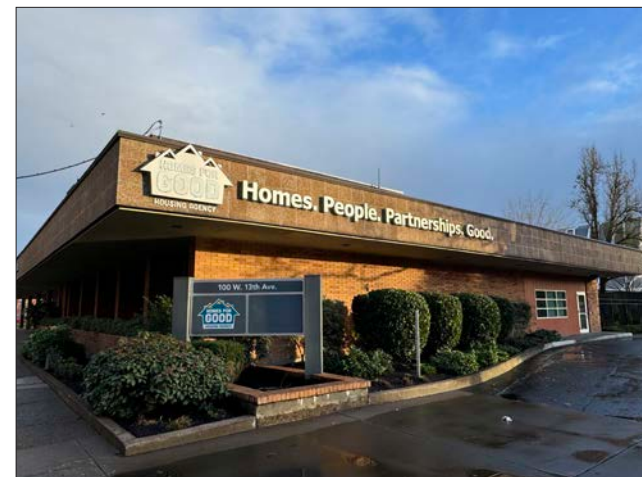
Exterior Building View
